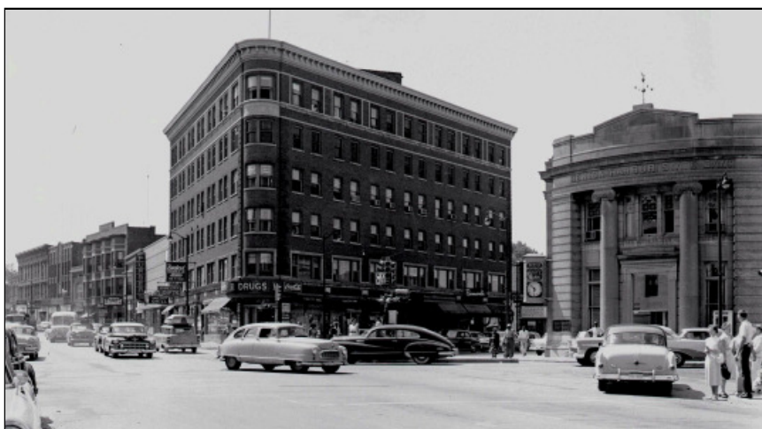
The Fidelity Building (center) and Benton Harbor State Bank, 1956.
